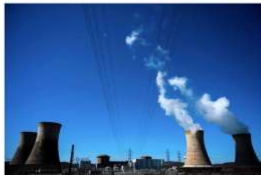
The Three Mile Island nuclear plant in Londonderry Township, Pa. Andrew Caballero-Reynolds/Agence France-Presse — Getty Images
